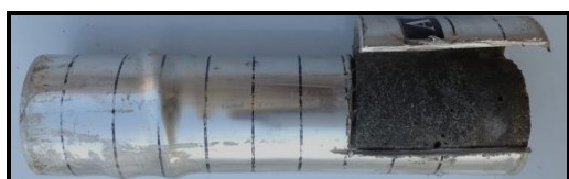
Plate (8) The smooth interface between aluminum tube and concrete
